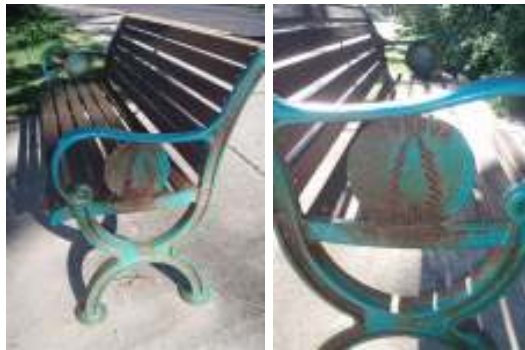
Above: the rust to the Cast iron “Tuross Head” seats on Tuross Boulevard
